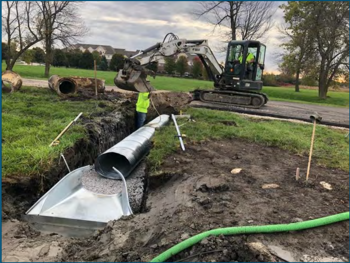
Figure 22: Typical Culvert Replacement
