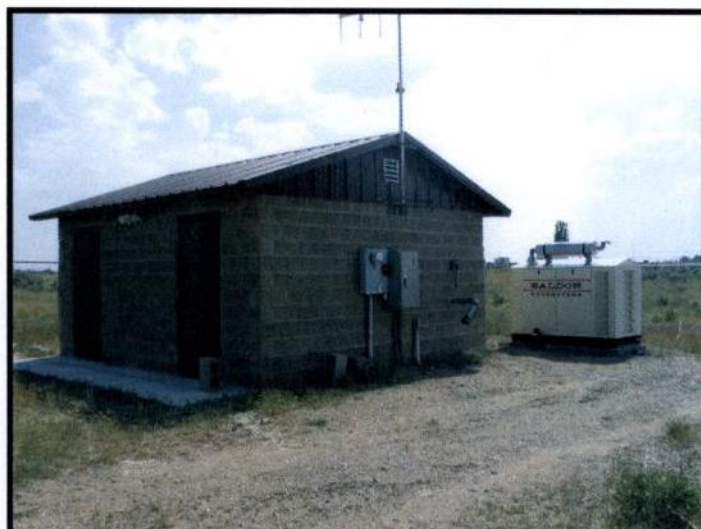
NEWTOWN WATER SYSTEM NO. 3 PUMPHOUSE — THOMAS LOOP
